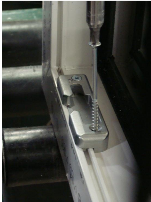
Figure 28: Replacing tilt & turn keeper screw to anchor sill
