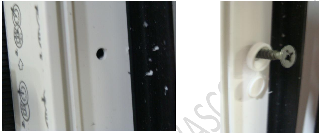
Figure 26: Installation hole (left), and with screw and cover (right)
